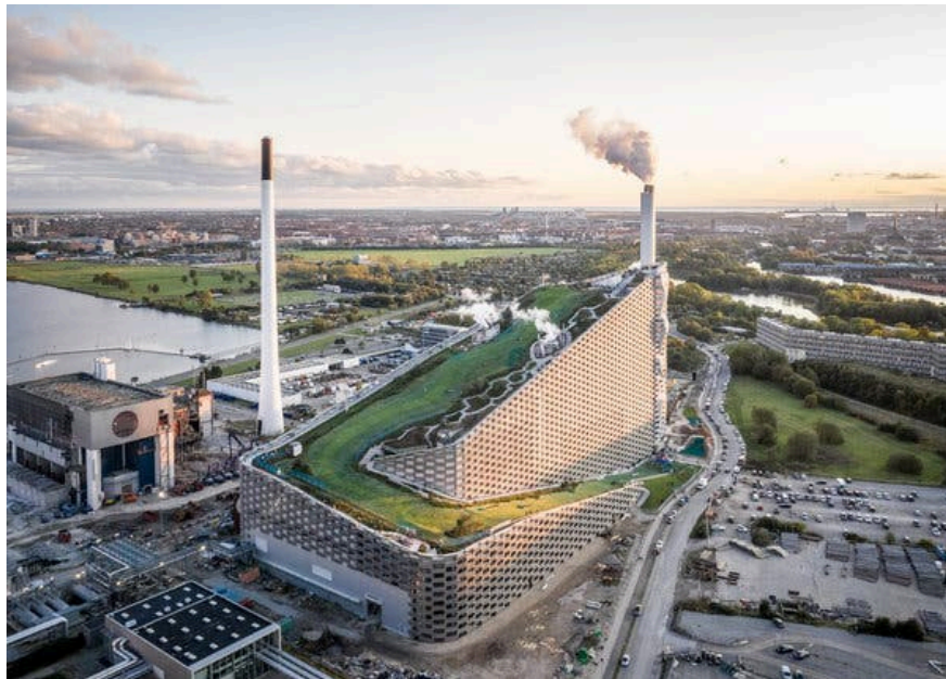
Figure 8. Amager Bakke incinerator in Copenhagen, Denmark (de Valence, 2019)
